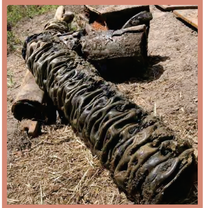
Original bursting head crumpling rather than splitting the existing pipe.
